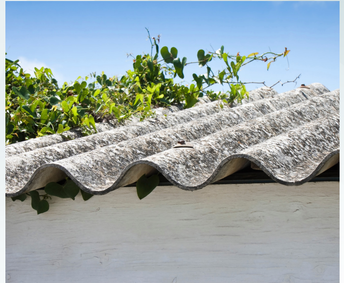
Traditional asbestos roofing sheet.
